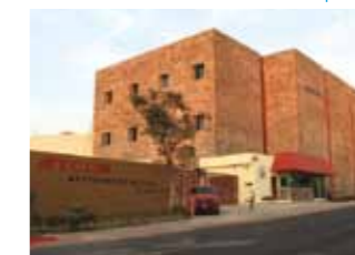
★ Cuernavaca Factory, Mexico MAYEKAWA DE MEXICO, S.A.DE C.V.
